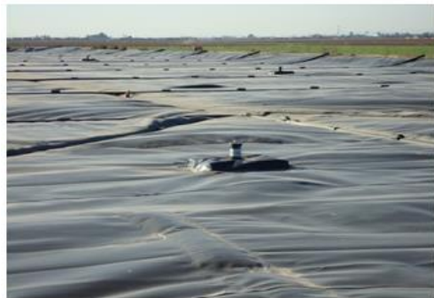
Covered Lagoon Digester
