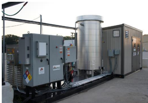
BIO CNG System CNG Pumps
